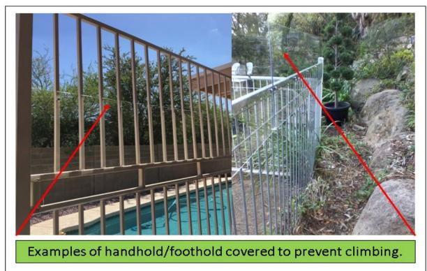
If the enclosure is constructed of chain-link, lattice, mesh, or any other similar material the openings must measure less than 1<sup>3</sup>/<sub>4</sub>" (measured horizontally)
