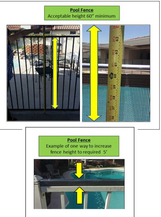
The exterior side of the fence is free of footholds and handholds. The Life Safety Inspector will look around the area and measure 3' from the fence to identify any potential items that could be used as a handhold / foothold or affect the height of the fence such as a change in landscaping.
